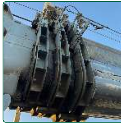
Shimming and Alignment
