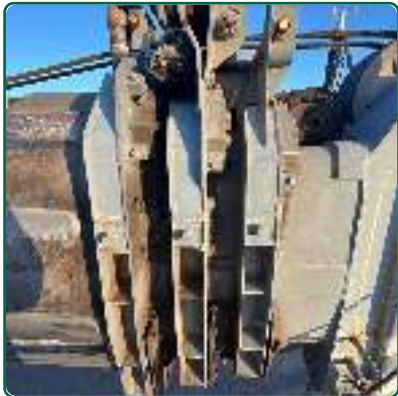
Shimming and Alignment
