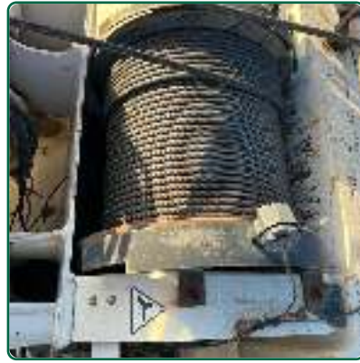
Winch Condition & Oil Level
