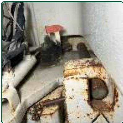
Counterweight Attachment - Security
