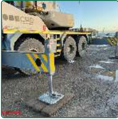
Outrigger Hazard Striping
