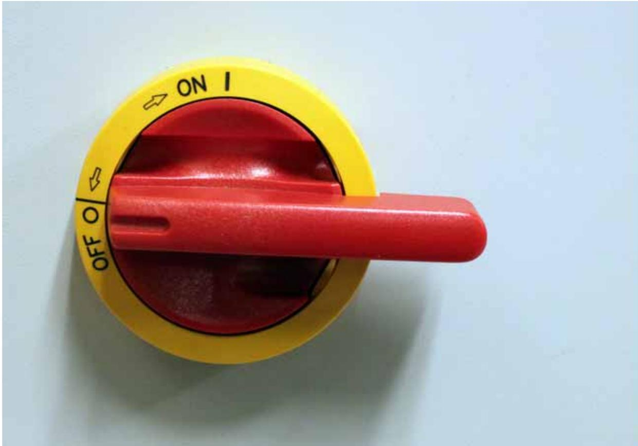
*Figure 4-1. Main Disconnect Switch*
